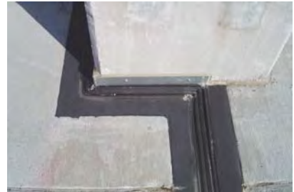
Factory pre-fabricated directional sections are recommended.
